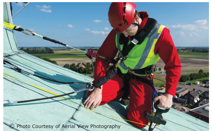
© Photo Courtesy of Aerial View Photography KT815 RAD Work Positioning
